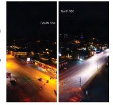
"The new lamps are also all 'Dark Sky compliant,' which is important to the City," says Pierotti. "The lamps we have installed have zero 'up-light.' They have very tight specifications for backlight and glare as well, plus we can install backside and side shields upon member request if members experience any glare through their home windows."
