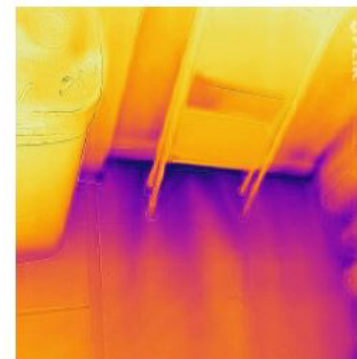
Air infiltration at bottom of kitchen wall in pantry where it shares with garage wall.
