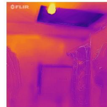
Attic accesses in master bedroom closet
