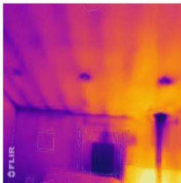
Air leakage at living room can lights and gas stove flue
